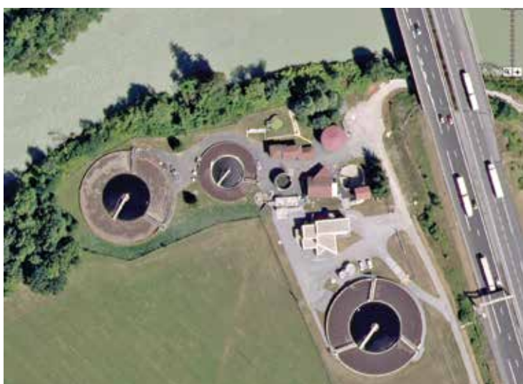
La station de Bellecombe
